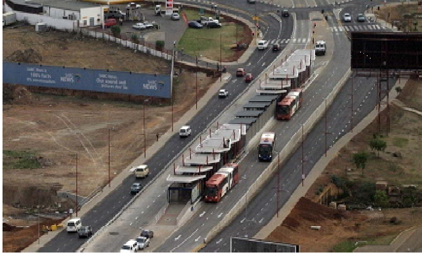
Figure 2: BRT station in Johannesburg with two substops
