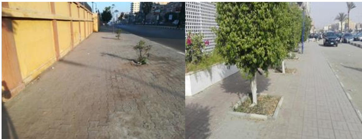
Figure 10. Trees positioned in the middle of footpath reduce clear space available for pedestrians: Al Azhar (left) and Hosary (right).
