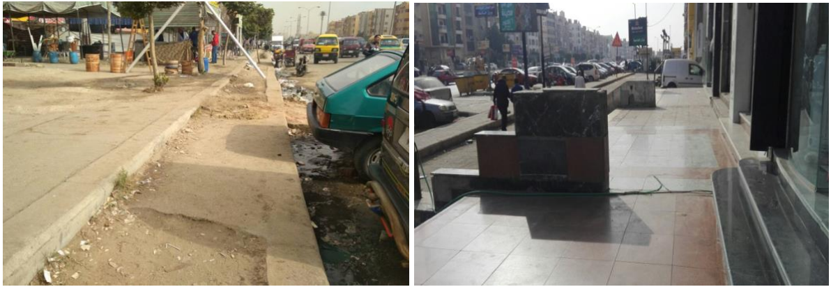
Figure 9. A lack of consistent design guidelines has resulted in frequent height differences, forcing pedestrians to walk in the carriageway: Emtedad Al Central (left) and Hosary (right).
