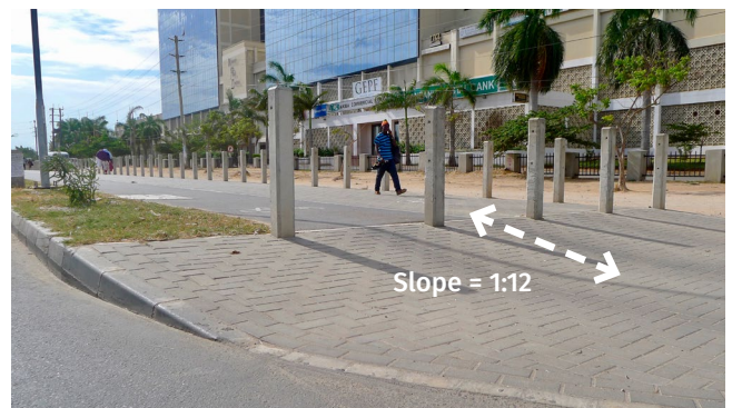
Figure 26. Where footpaths are ramped down to the level of the carriageway, the maximum ramp slope is 1:12.
