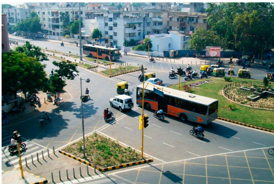
Figure 83. Squareabout intersection with two-phase signal cycle permitting BRT and mixed traffic turning movements together.
