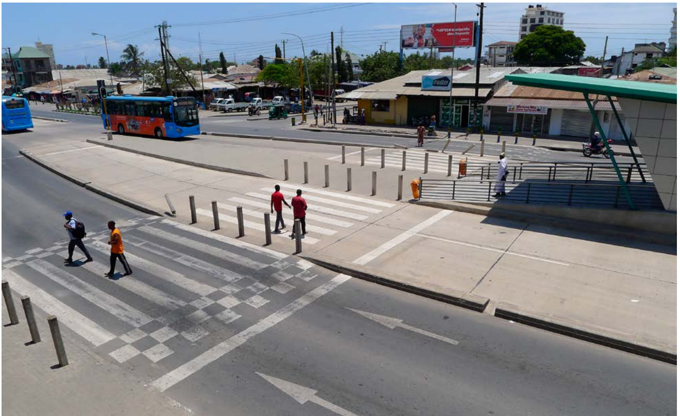
Figure 32. A tabletop crossing provides safe access to a BRT station.
