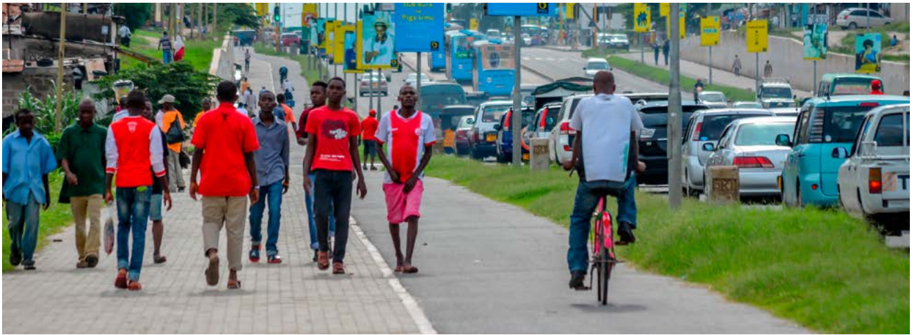
Figure 35. This cycle track is physically separated from the carriageway, has a smooth surface material, and is wide enough for cyclists to overtake one another.
