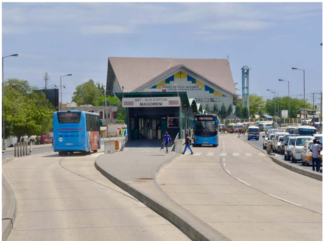
Figure 50. Passing lanes can increase the passenger capacity of a BRT system by allowing express buses to overtake local buses at certain stations.
