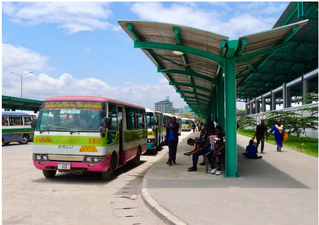
Figure 45. High-quality matatu/bus terminals offer protection from sun and rain, seating, and universal access.
