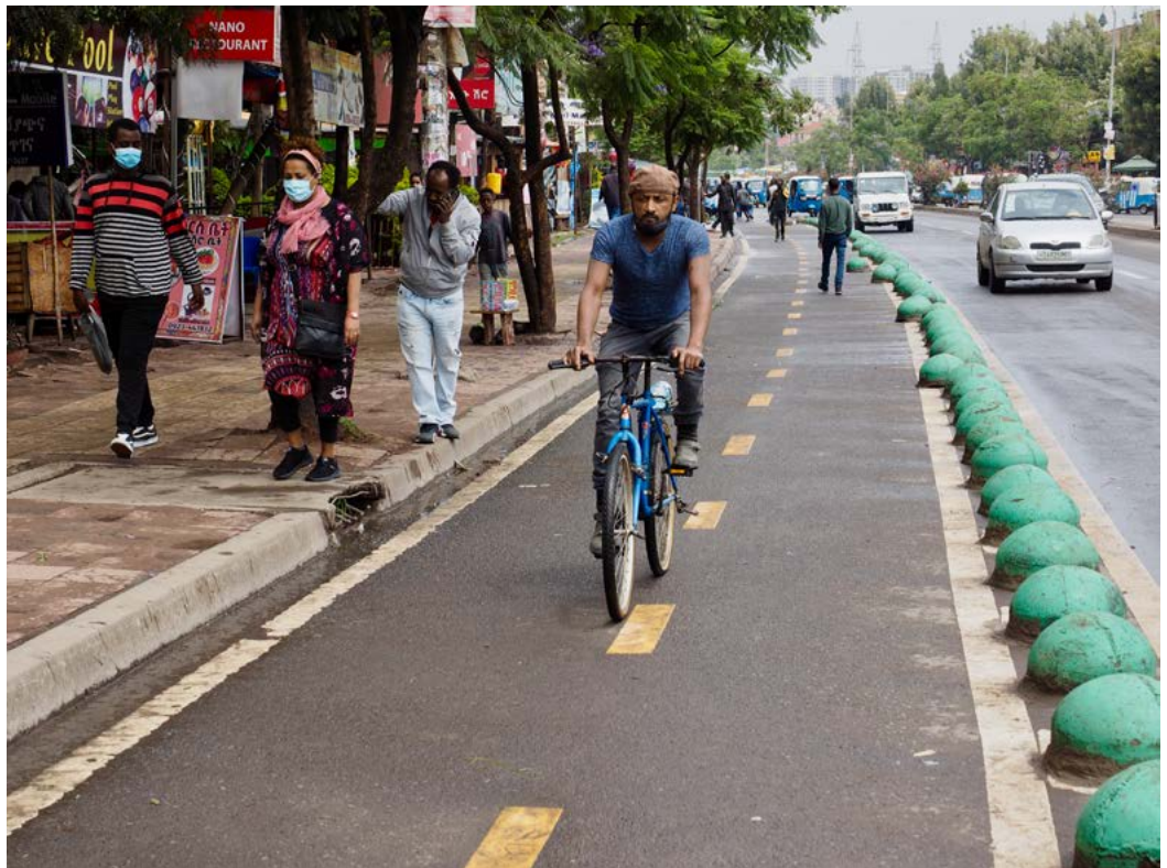
Figure 40. Part of an oversized carriageway can be re-purposed as a cycle track. Physical separators protect cyclists from motor vehicle traffic.
