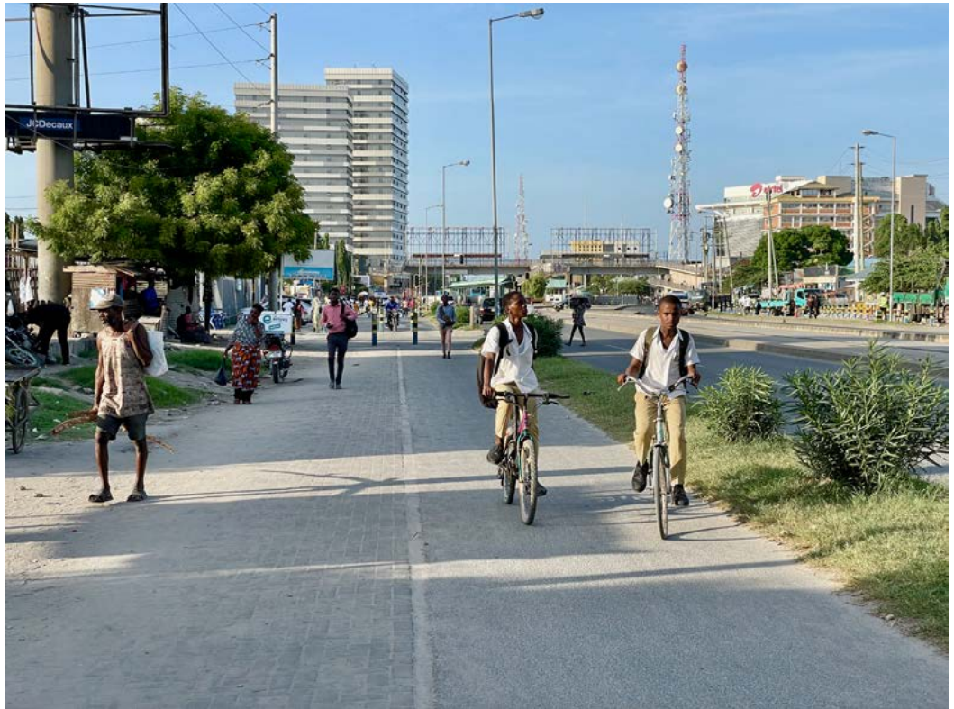
Figure 39. Newly constructed cycle tracks should be physically separated from motor vehicle traffic and raised +150 mm above the carriageway.
