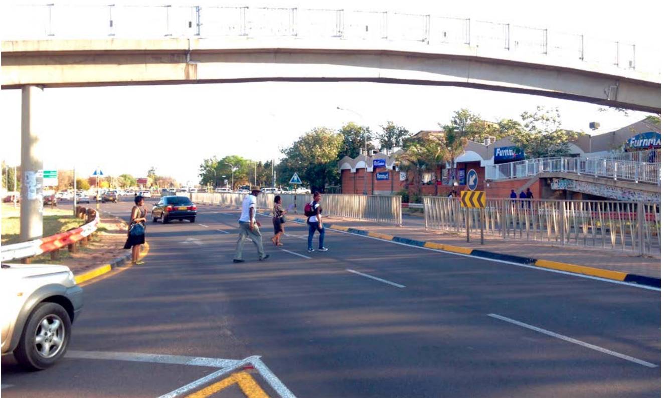
✘ Figure 33. Footbridges often represent a wasted investment. When presented with a choice, pedestrians prefer to cross at street level.
