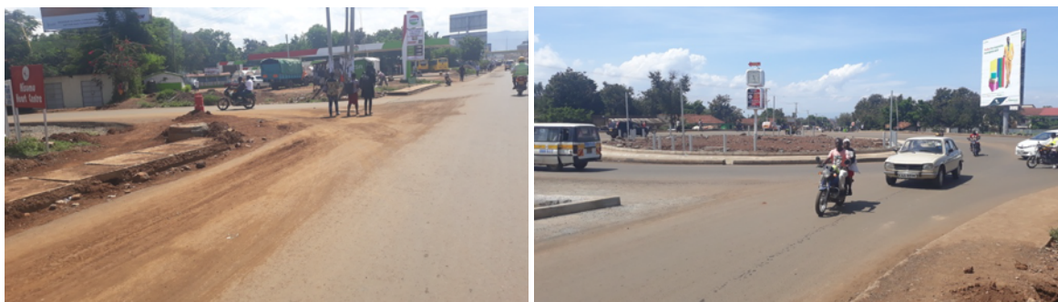
Figure 58: Wide turning radii at intersections encourage drivers to move at high speeds, thus endangering NMT users.
