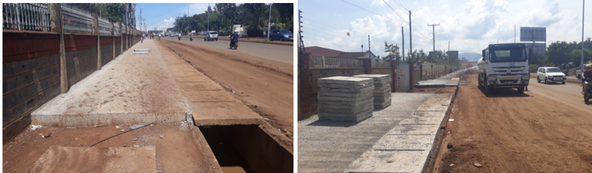
Figure 57: The Kenyatta Highway project includes concrete footpaths along some stretches. However, the design does not incorporate universal access or tree cover.
