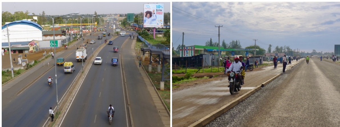
Figure 56: While service lanes on Nairobi Rd sometimes function as shared spaces, most stretches lack traffic calming elements that would make them safe for walking.
