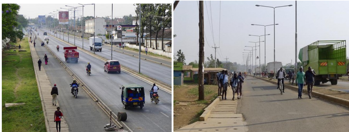
Figure 15: Wide shared lanes for pedestrians and cyclists along Nairobi-Busia highway. The NMT facilities are often encroached by motor vehicles, introducing safety risks for pedestrians.
