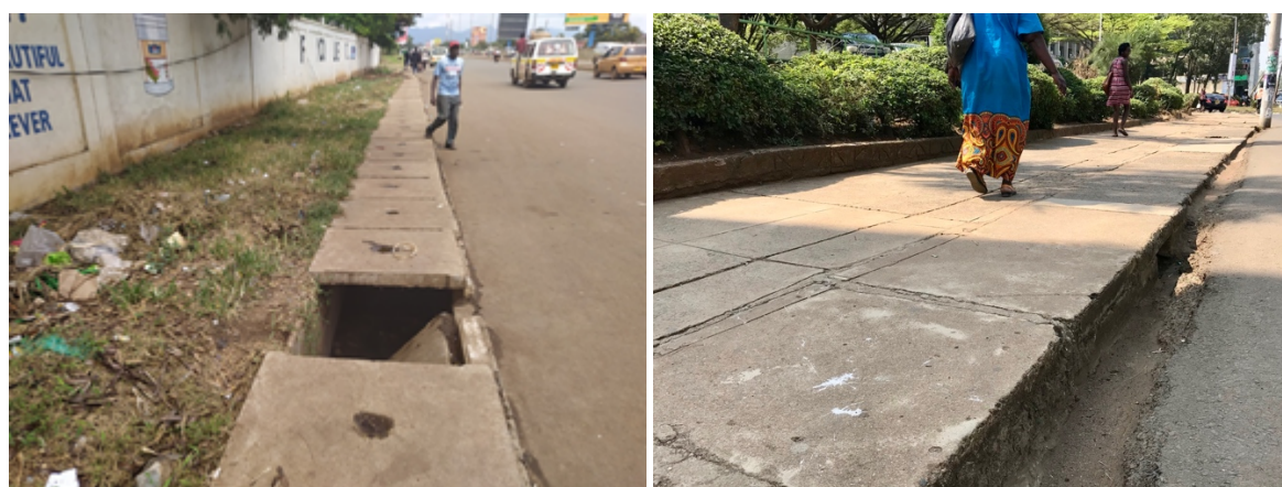
Figure 87: Loose drain covers make for a poor walking surface (left). A well-finished footpath on top of a major stormwater drain provides a comfortable walking surface (right).
