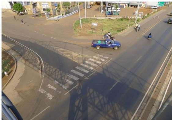
Figure 18: Wide turning radii at intersections encourage speeding by vehicles, thus making it unsafe for pedestrians to cross the road.
