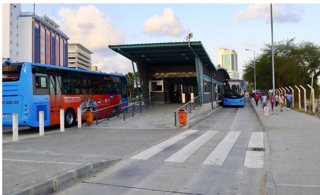
Figure 11. Integration of BRT with wide footpaths in Dar es Salaam.
