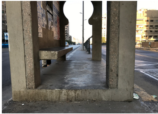
Figure 28. Bus shelters recently installed in Cairo have a large step, thereby compromising access for persons with disabilities. In the new communities, shelters are often absent.
