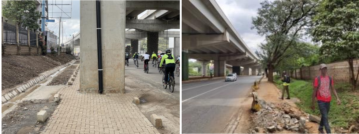
Figure 13. Some footpaths along the A8 have been reinstated, but the alignment of the footpaths did not account for the presence of Expressway columns.
