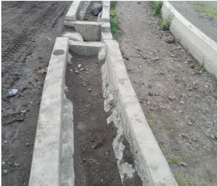
Figure 39. Kality-Tulu-Dimtu cycle track under construction.
