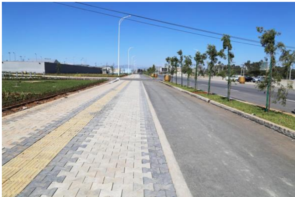
Figure 43. Bole Airport to Goro, under construction.
