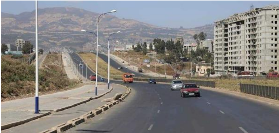
Figure 35. Haile Garment-Furi roundabout cycle track under construction
