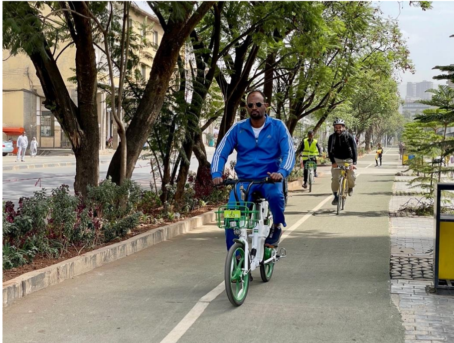
Figure 40. Mezegaja-Meskel Square street refurbishment project.
