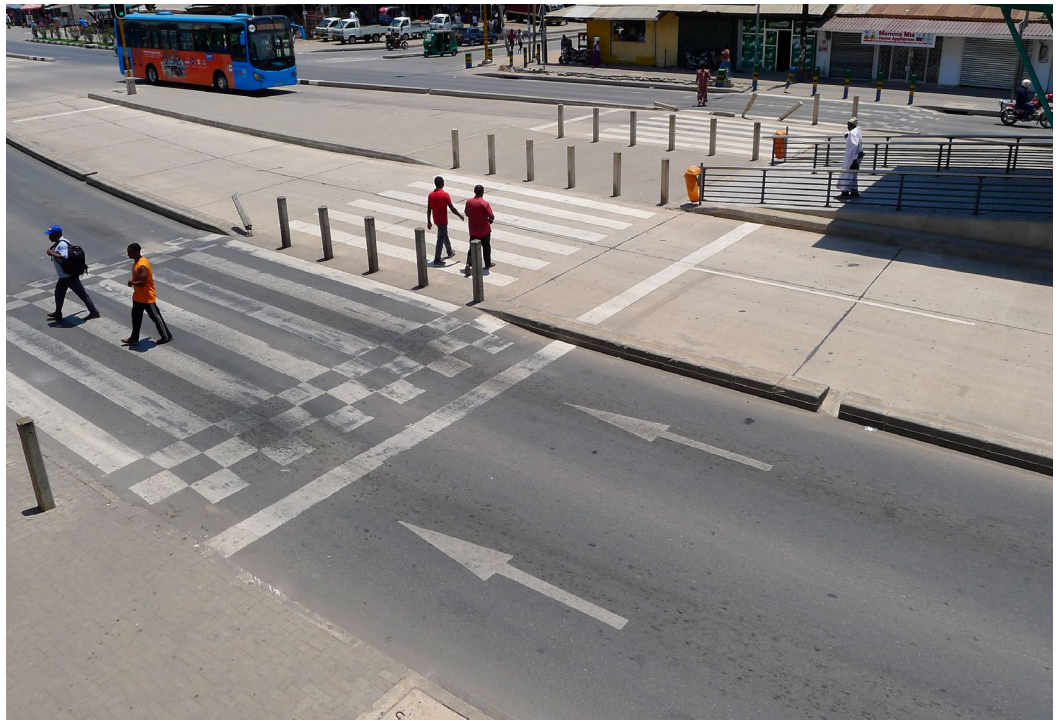
Figure 32. A tabletop crossing provides safe access to a BRT station.
