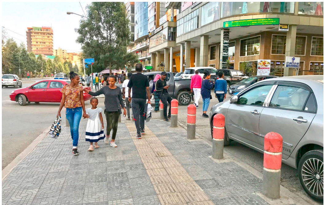
Figure 24. Bollards prevent vehicles from parking on footpaths.
