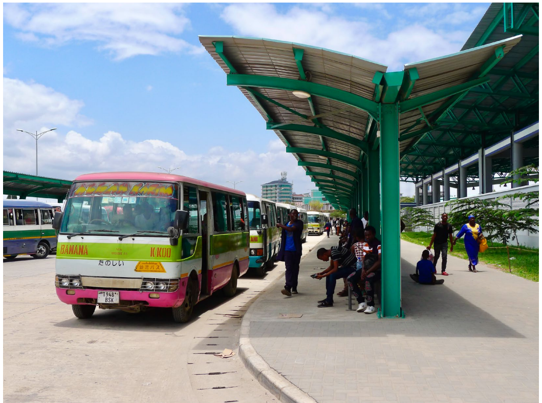
Figure 46. High-quality bus terminals offer protection from sun and rain, seating, and universal access.
