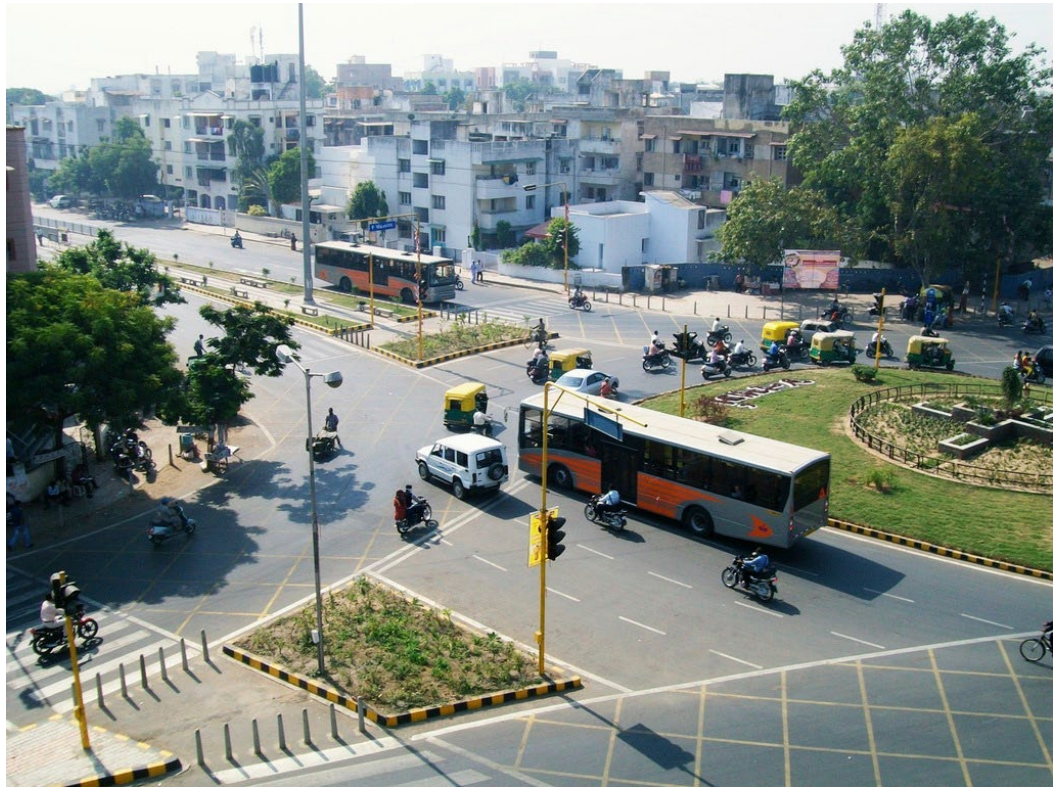
Figure 81. Squareabouts allow for two-phase signal cycles, which can reduce total signal cycle times in intersections with median BRT lanes.
