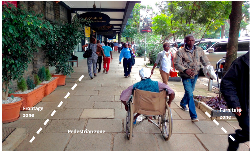
Figure 19. Footpaths designed per the zoning system provide uninterrupted walking space for pedestrians. The pedestrian zone should have at least 2 m of clear space.
