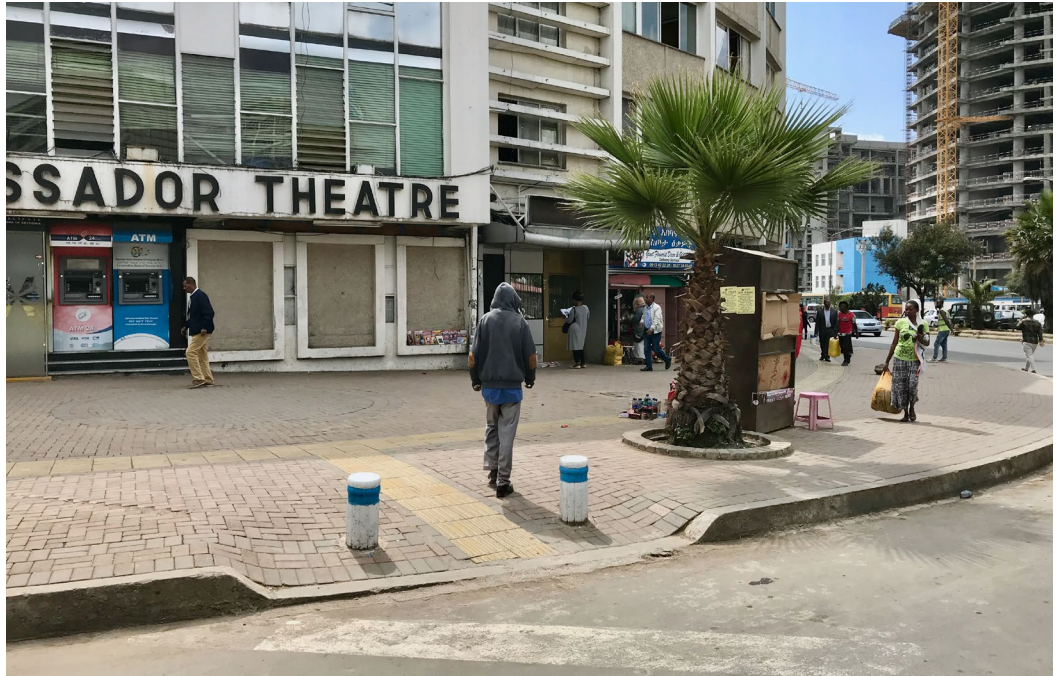
Figure 26. Footpaths should ramp down to the level of the carriageway, with a maximum ramp slope of 1:12.
