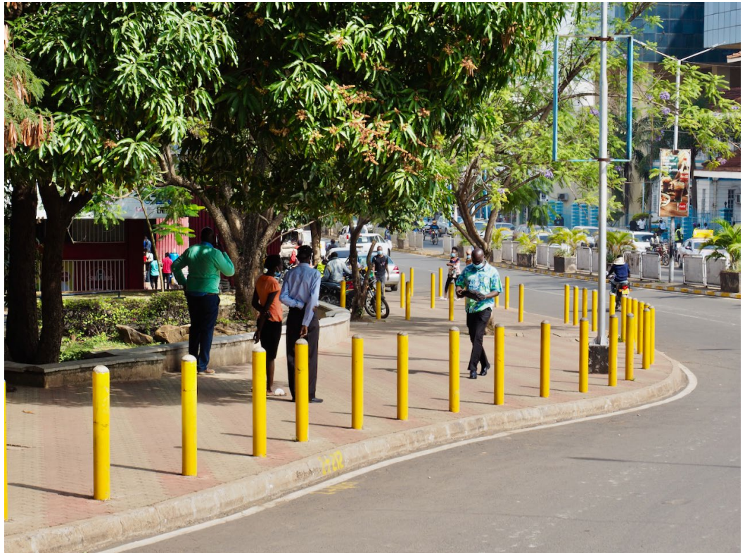
Figure 25. Footpaths placed below the carriageway often experience water-logging. Footpaths should be raised +150 mm above the carriageway.
