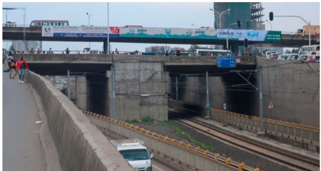
Figure 83. Underpass and bridge.
