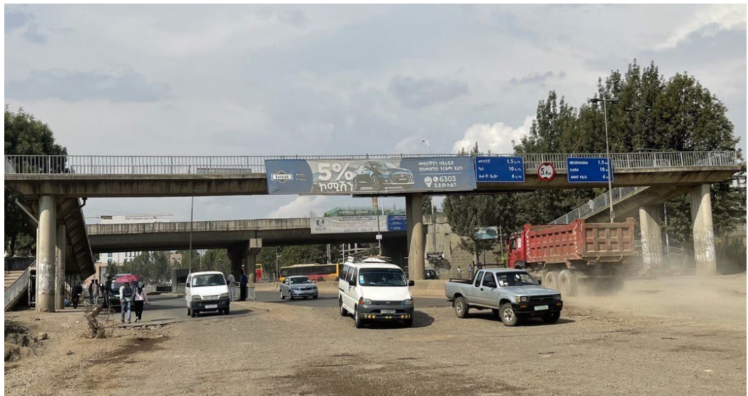
Figure 33. Pedestrian footbridges create longer routes, leading pedestrians to risk crossing at the shortest distance.
