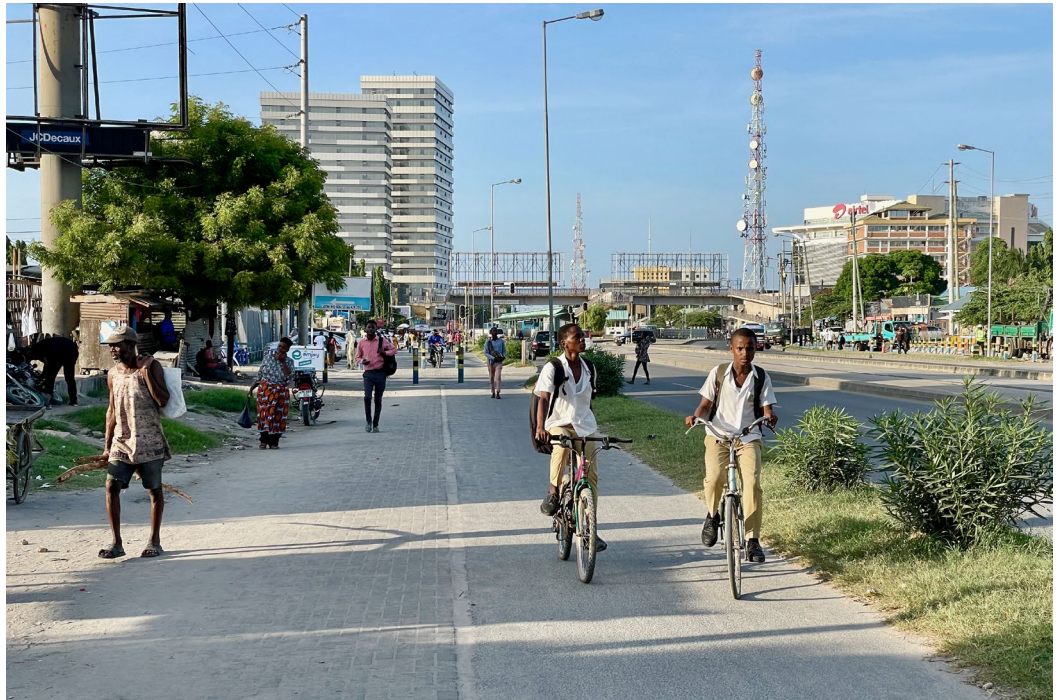
Figure 35. Newly constructed cycle tracks should be physically separated from motor vehicle traffic and raised +150 mm above the carriageway.
