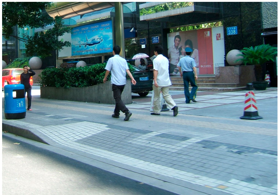
Figure 28. Treatment of property entrances. Footpaths should remain at the same level at property entrances and small side streets, with ramps for vehicles, in order to improve convenience for pedestrians and maintain universal access.
