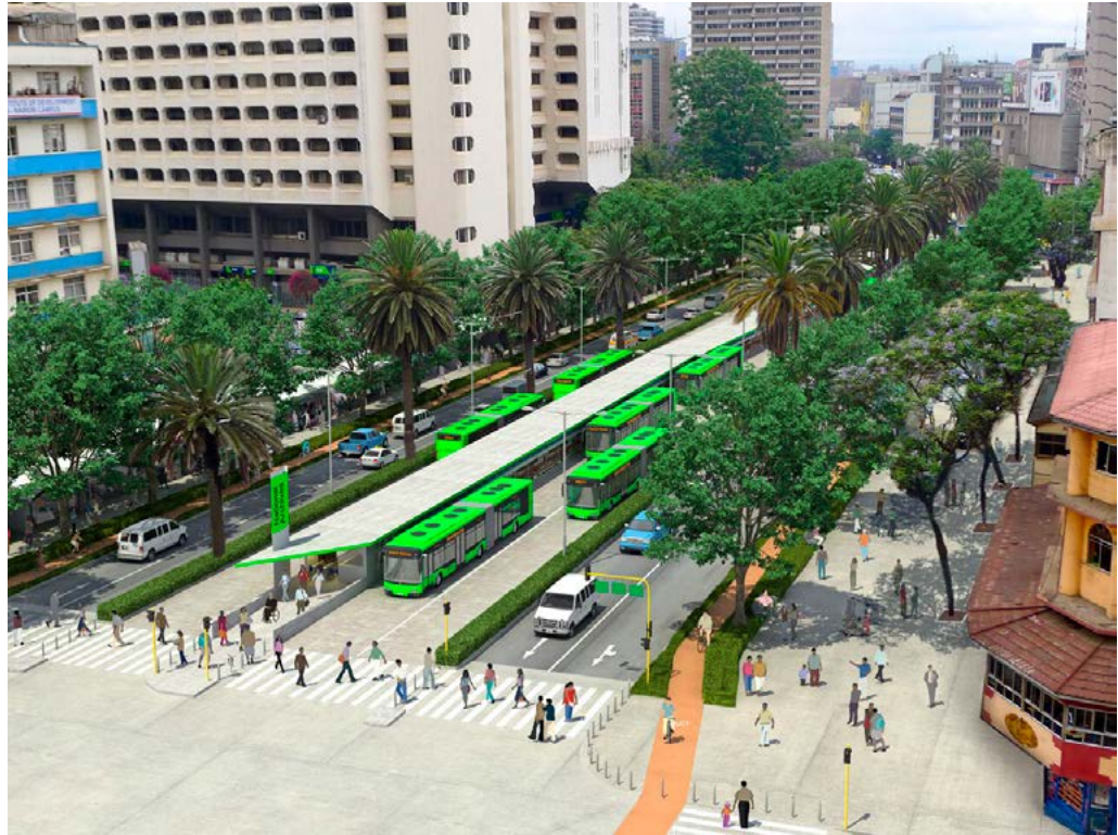
Figure 8. High-quality BRT corridors incorporate dedicated bus lanes, central station platforms, and good NMT access.
