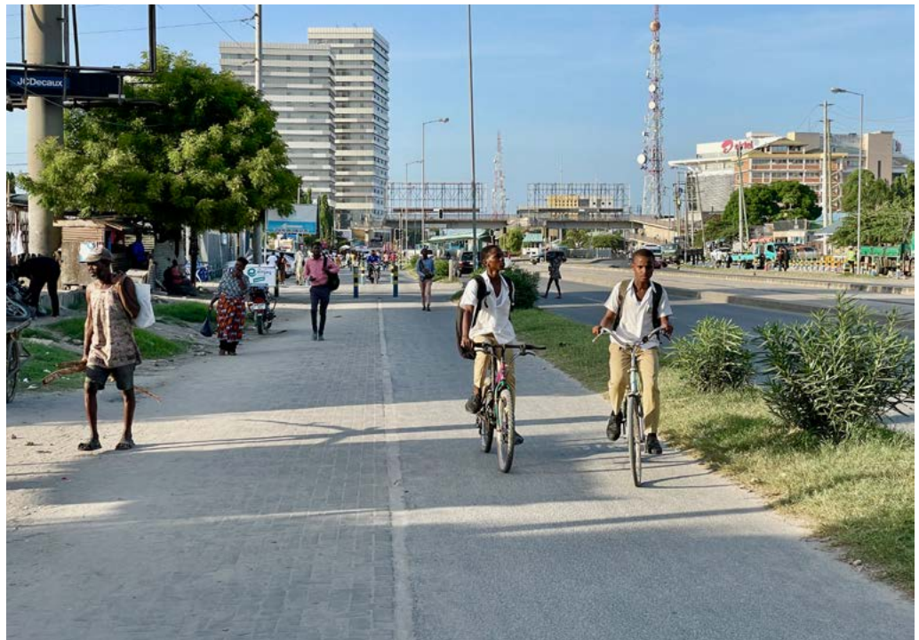
Figure 14. Cycle track in Dar es Salaam.
