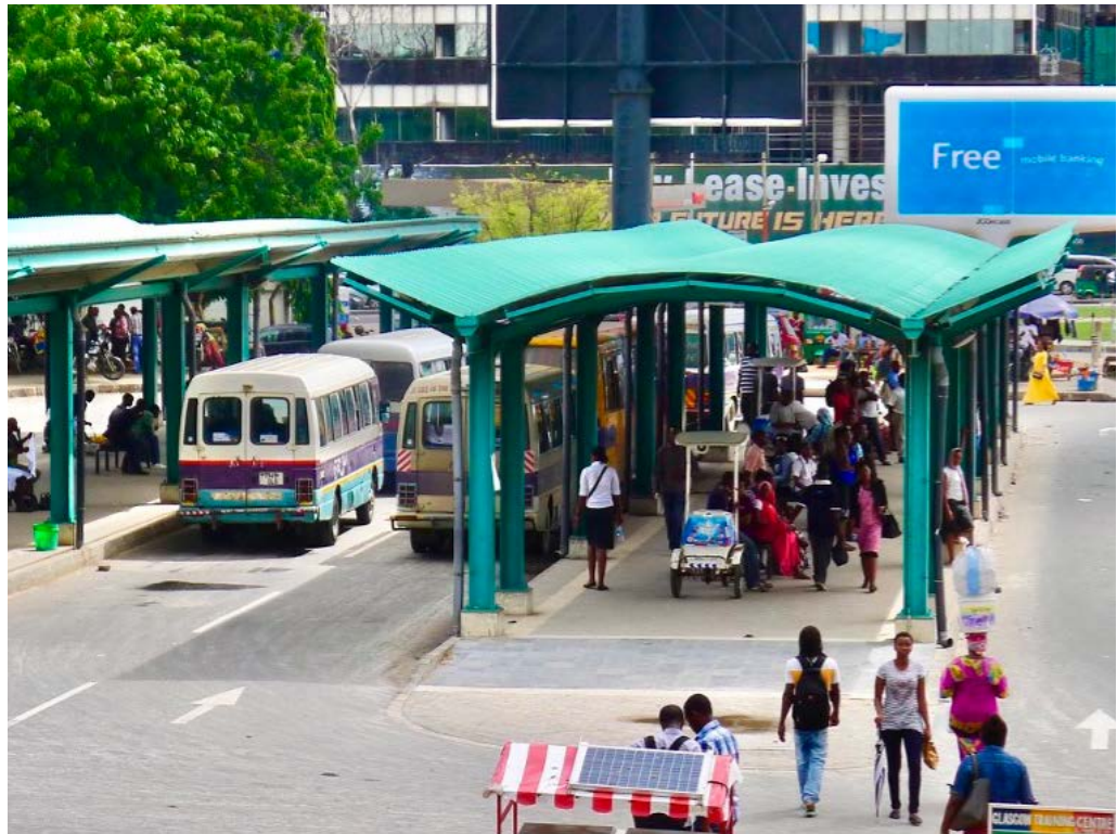
Figure 12. Well-designed bus terminals offer comfortable waiting areas for passengers.
