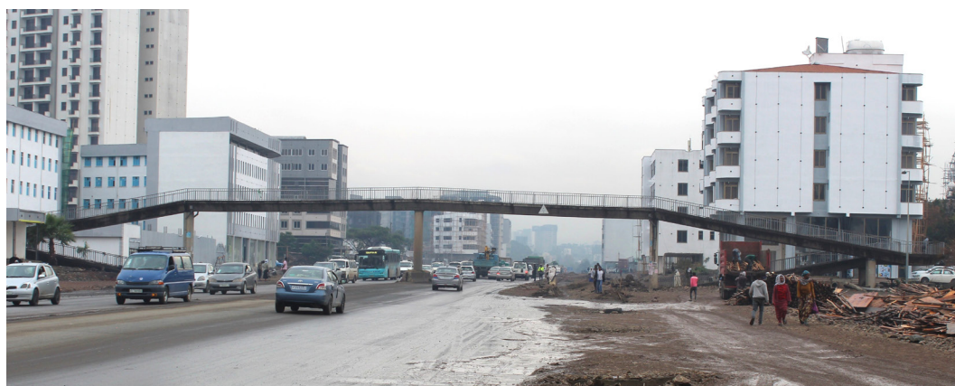
Figure 12. Pedestrian crossing bridge across the former ring road from Lebu- German square, which is under maintenance at present
