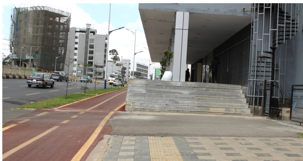
Figure 2. The steps in the arcades and walkways limit accessibility.
