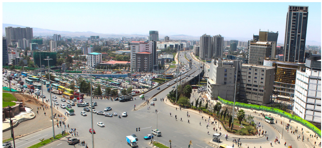
Figure 13. The roundabout at Diaspora Square has been converted into a signalised intersection. Adequate mobility still needs to be worked out to enhance safe crossing.
