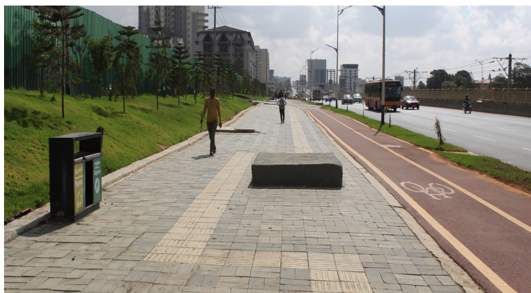
Figure 22. Manhole obstructing the footpath continuity and a right-angled tactile lane detour failing to provide smooth, accessible mobility for visually impaired pedestrians.
